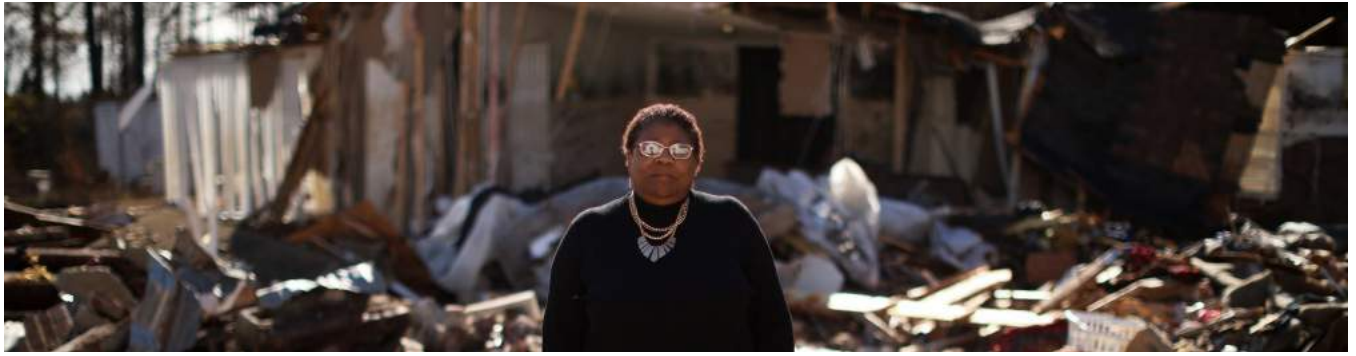
Linda Worsley outside her Princeville home, which was demolished after being damaged in a flood caused by Hurricane Matthew. Photos by Travis Dove.
