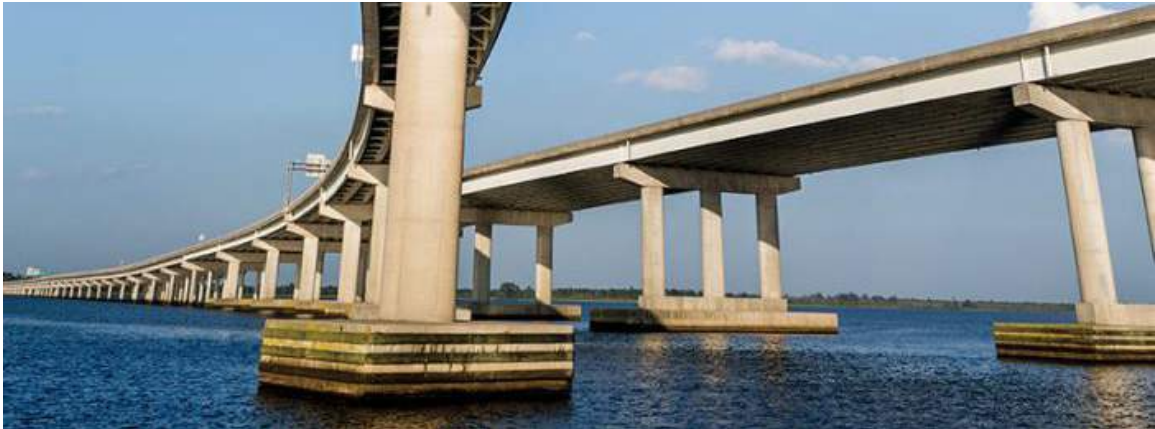
Since 1999, the Neuse River Bridge has carried drivers up and over the Trent and Neuse rivers. PHOTOS BY CHARLES HARRIS
